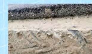
■ 固化剂稳定土基层 Curing agent stabilizes the soil base
